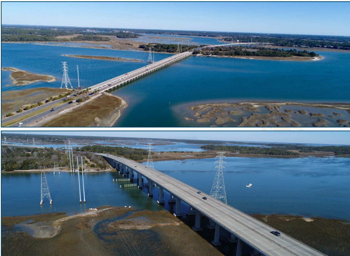
Figure 1-2 US 278 over Mackay Creek (top) and US 278 over Skull Creek (bottom)
