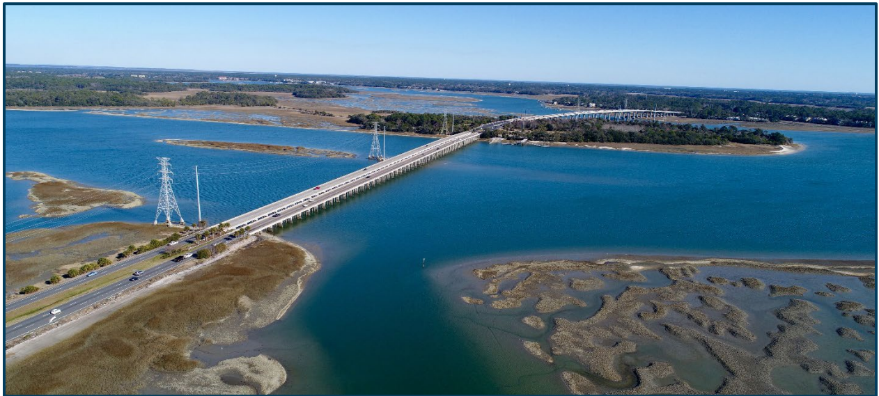
Figure 2-1: Mackay Creek and Skull Creek bridges
