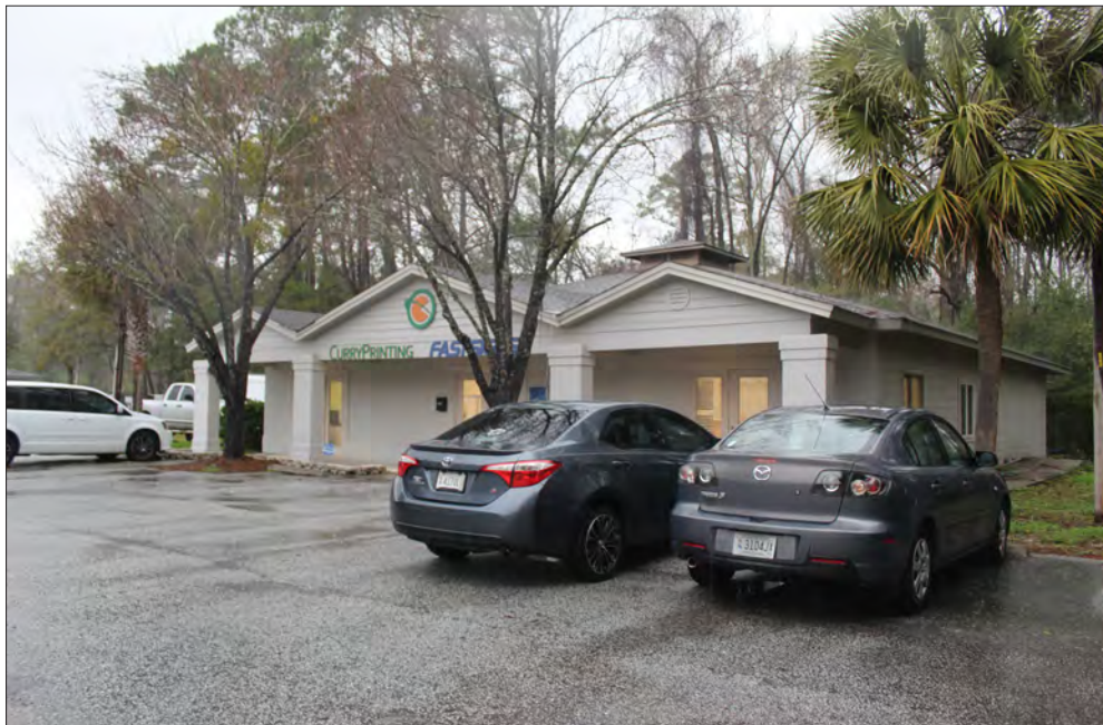
23b. Commercial office building at 157 William Hilton Parkway, Facing Northwest
