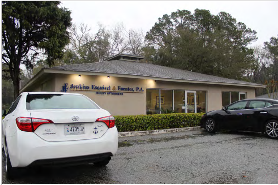
23a. Commercial office building at 155 William Hilton Parkway, Facing Northeast
