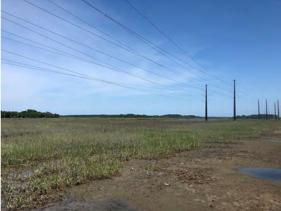
Photo #21 CATA, north of US 278 (32.218338, -80.762809) Figure 7
